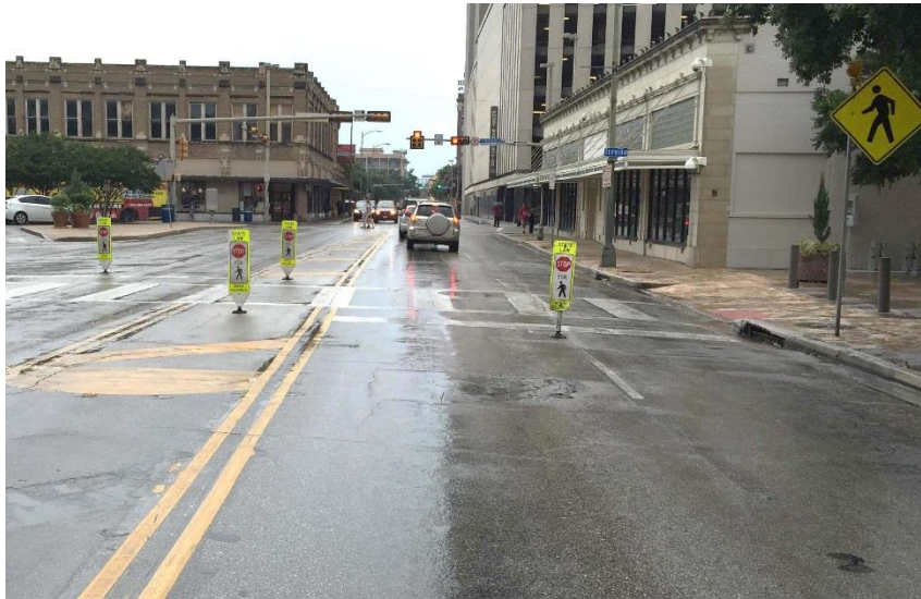
58 59 Figure 1. An incomplete gateway that resulted from a combination of narrow lane width 60 and drainage issues.
