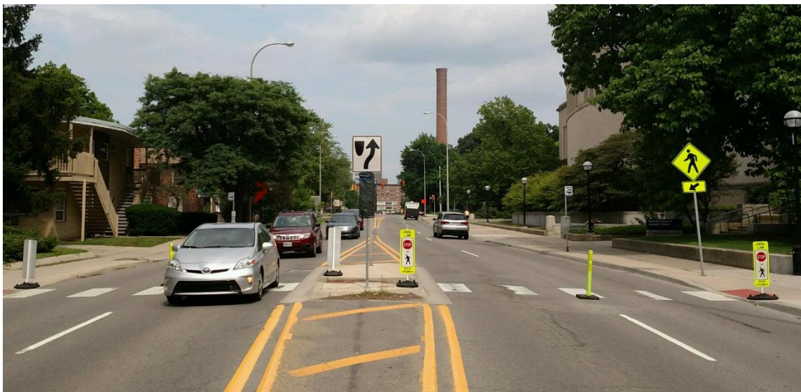
77 78 Figure 2. The Gateway condition at Huron with the signs placed on top of the curbs. 79
